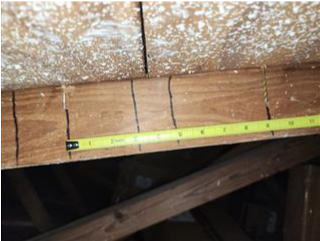
Roof Deck Attachment Spacing
