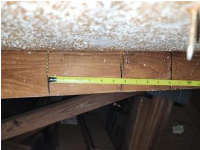
Roof Deck Attachment Spacing
