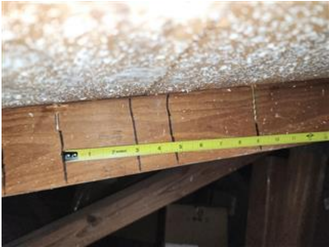
Roof Deck Attachment Spacing
