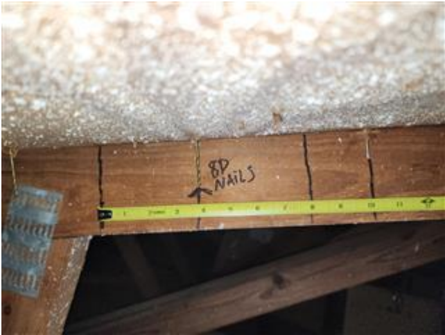
Roof Deck Attachment Spacing
