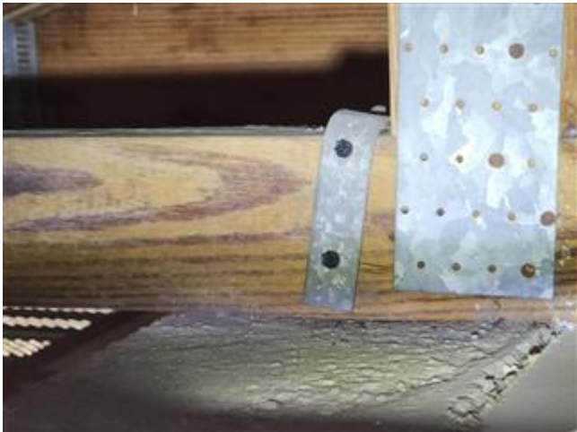
Truss Cord Attachment Single Wrap
