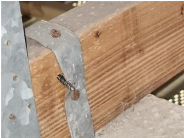
Truss Cord Attachment Single Wrap
