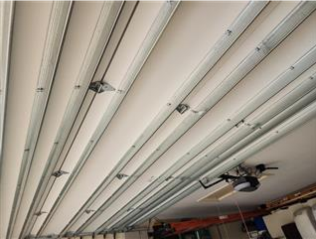
Interior Garage Door
