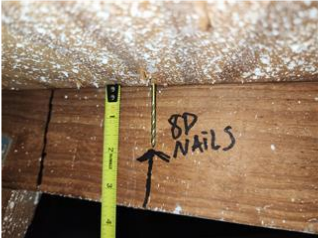
Roof Deck Attachment
